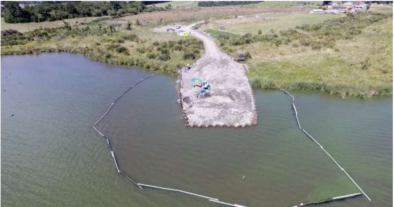
Figure 13. Progress at the Arawhata boat ramp. Photo taken 17 February 2021.
